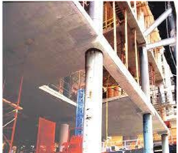
Fig. 2. Large opening in flat slab [1]
