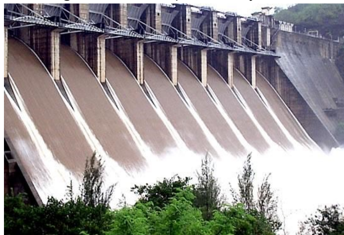
Fig. 2. Spillway of Karjan Dam under operation
